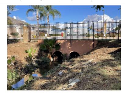
Photo 14: View facing north of two culverts that run underneath Hemlock Ave at north/northwest property boundary of Parcel A.
