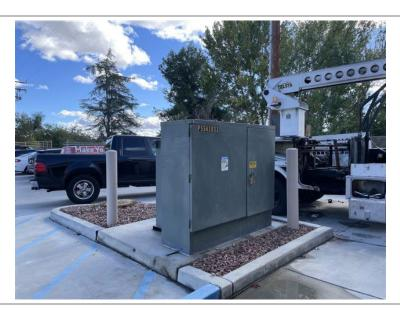
Photo 39: View of pad mounted transformer located in parking lot in Parcel E.
