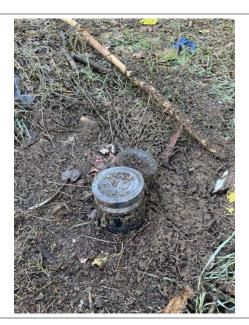
Photo 18: View of two black PVC pipes with rubber caps, likely sewer cleanouts, located at the south central boarder of Parcel A.
