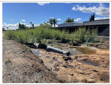
Photo 56: View of broken piping found in stormwater in Parcel Q.
