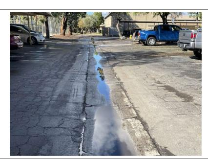
Photo 8: View facing west along the southern most street along the tennis courts. View of ponded stormwater typically observed throughout Parcel A from recent storm event.
