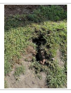
Photo 13: Close up view of a hole in ground/void in the vegetation adjacent to stormwater drainage culvert (see next photo) at north part of Parcel A.
