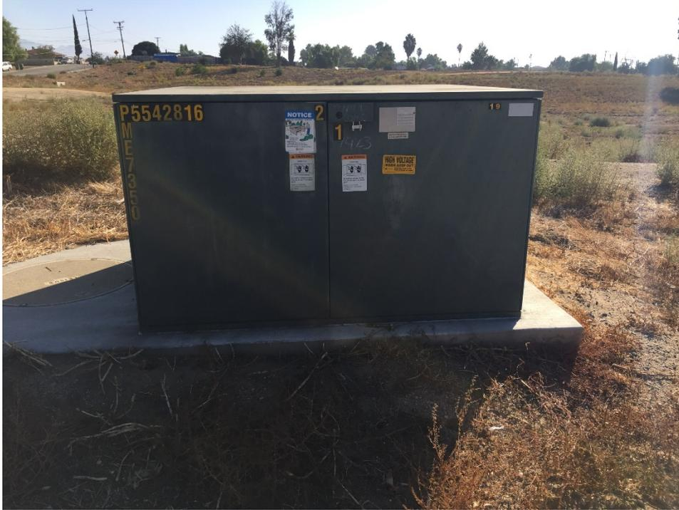
Photo 9: Second pad-mounted transformer along the western border of the Property.
