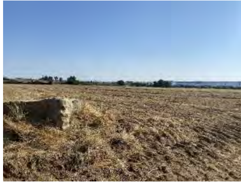
Photo 26: Looking southwest from Goya Avenue towards concrete debris at the Project Site along northern site boundary.
