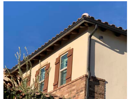
Example of Painted Downspouts Located at the Side of the Building
