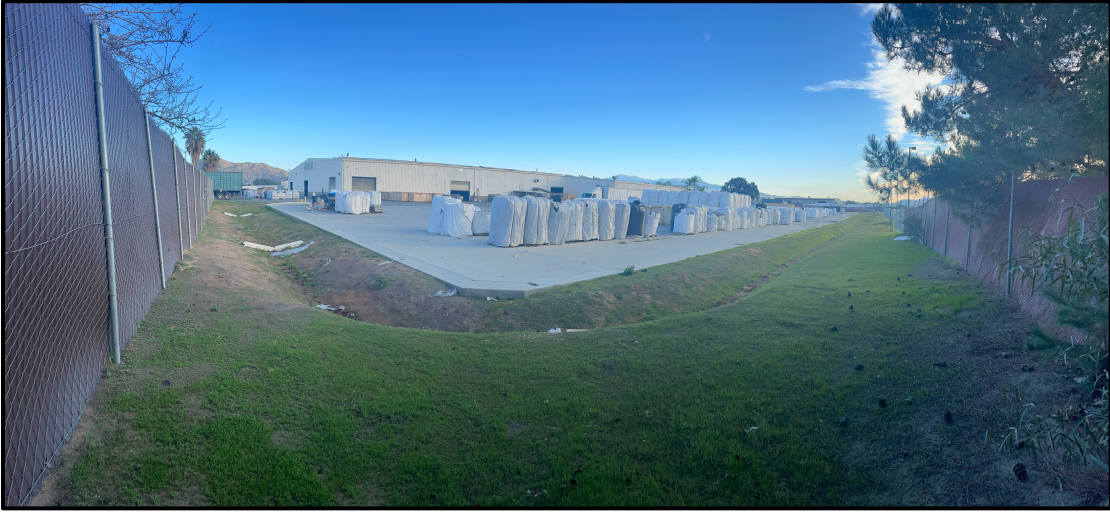
Plate 5.2-1: Overview of the project from the southwest corner, facing northeast.
