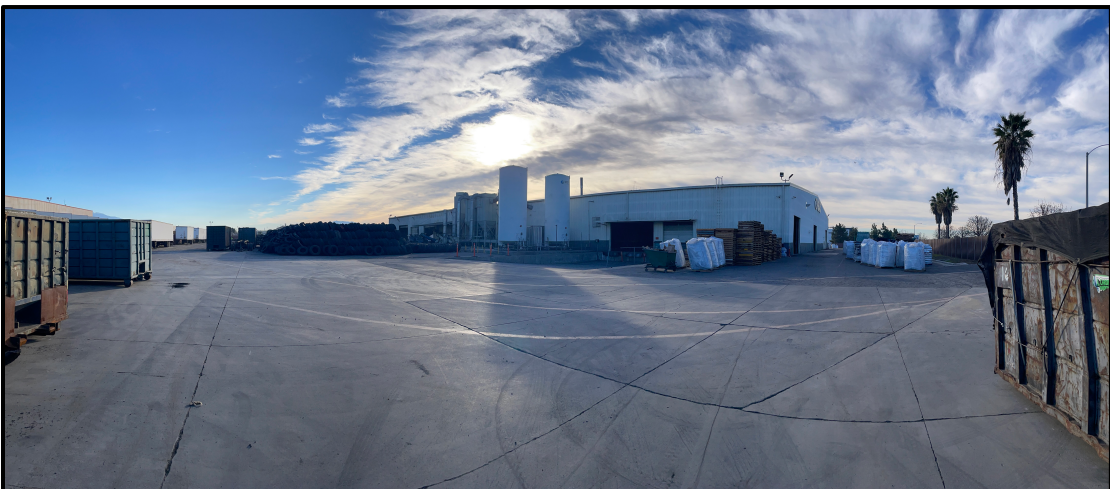
Plate 5.2-3: Overview of the project from the northwest corner, facing southeast.
