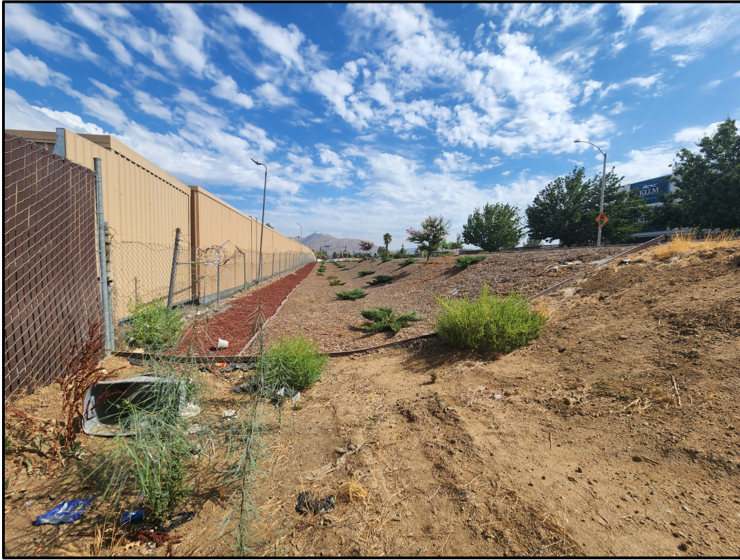
Plate 5.2–4: Overview of the off-site improvement area, facing north.
