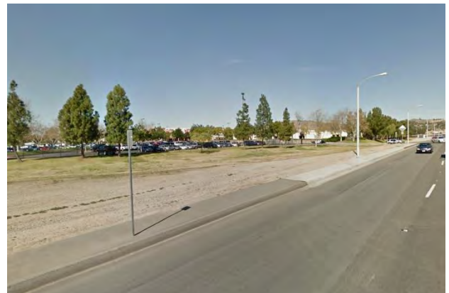
Incomplete sidewalks, often obstructed by street signage, are common along the Nason St Corridor.
