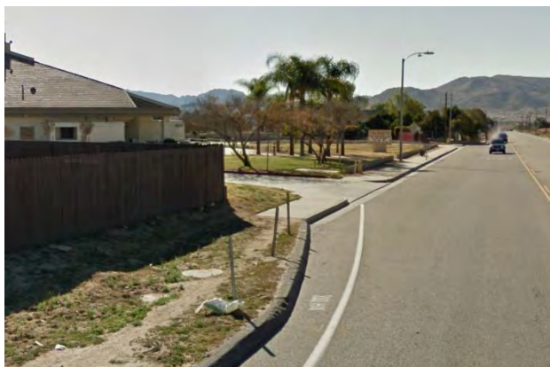
Incomplete sidewalk network: common at transitions between original rural development patterns and more recent development projects.
