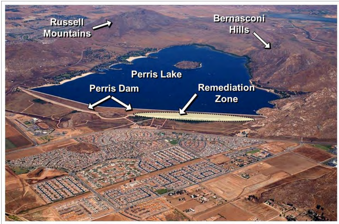
Figure 12-1: Perris Dam Construction Project 72
