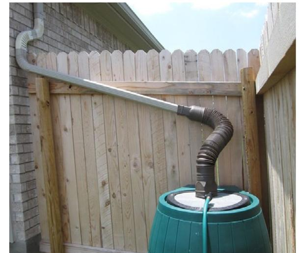
Rainwater harvesting can take the form of a greywater system (left) or a low-tech barrel in one's backyard that stores rain for a future dry day (above).
