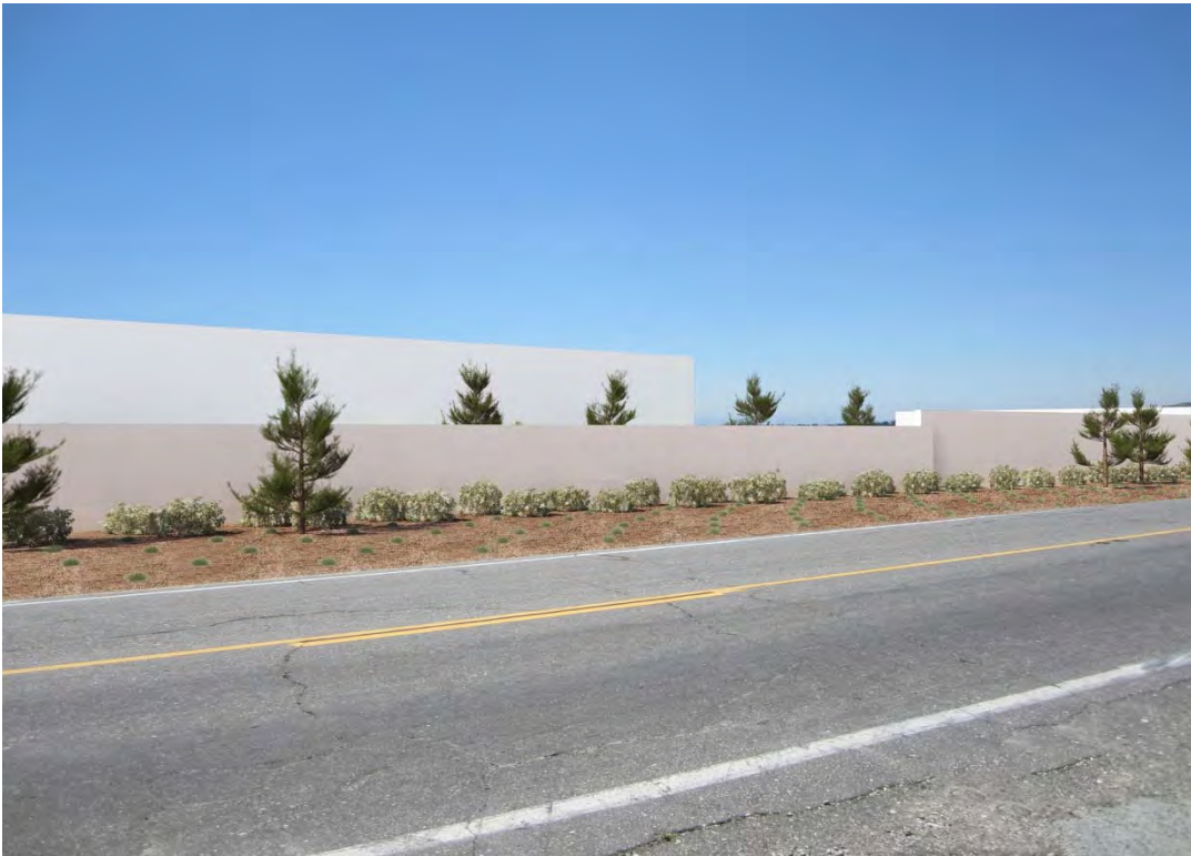
Gilman Springs Rd. View 5 at Installation
