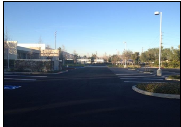
Figure 2 - CRC Parking Lot AFTER
