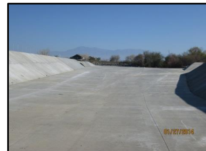
Upstream at the Channel Inlet
