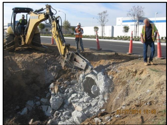
Construction of a culvert located south of the existing second lane on Cactus Avenue between Elsworth Street and Veterans Way, which will ultimately be widened to add a third lane to increase the level of service during peak traffic congestion times.
