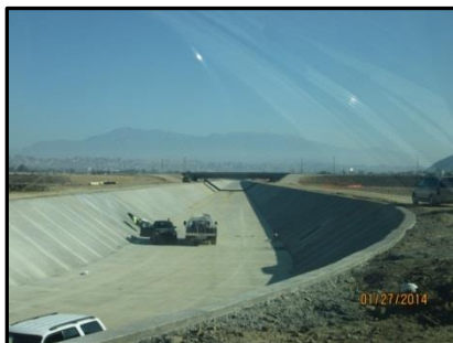
Looking East Upstream from the Channel Outlet
