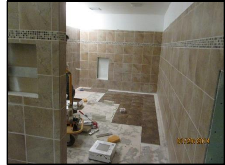
Tile Work: In Progress
