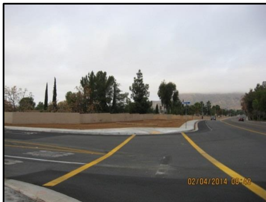
After: Completed Installation of ADA Compliant Access Ramp, Sidewalk and Roadway Realignment at the Southwest Corner of Indian Street and Manzanita Avenue
