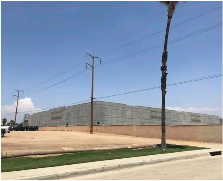
View of Adjacent Bldg Under Construction
