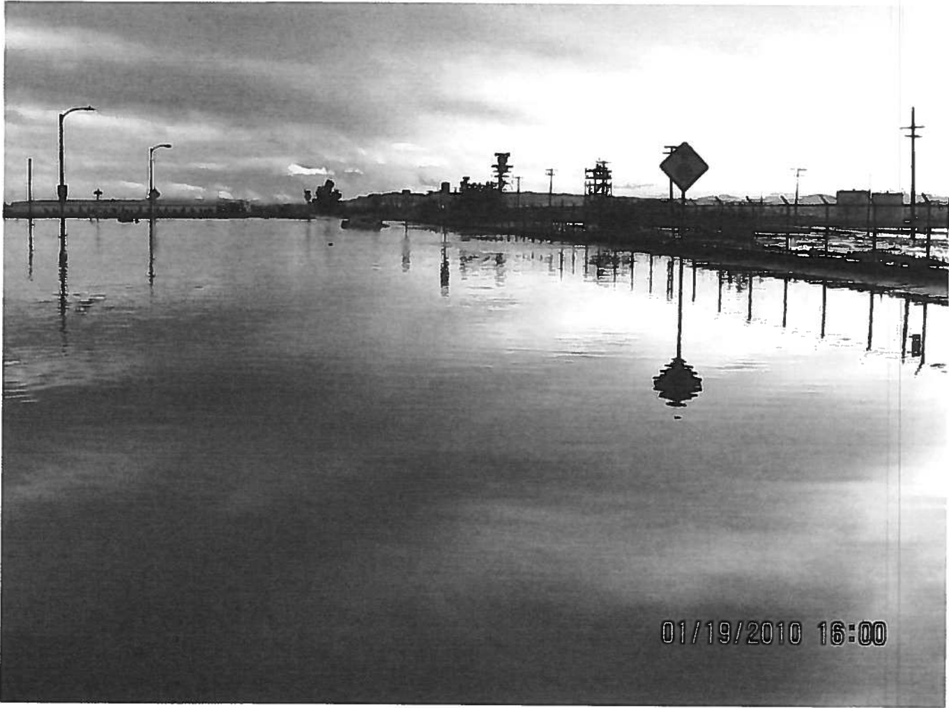
Flooding along Heacock Street between Gentian Avenue and Iris Avenue
