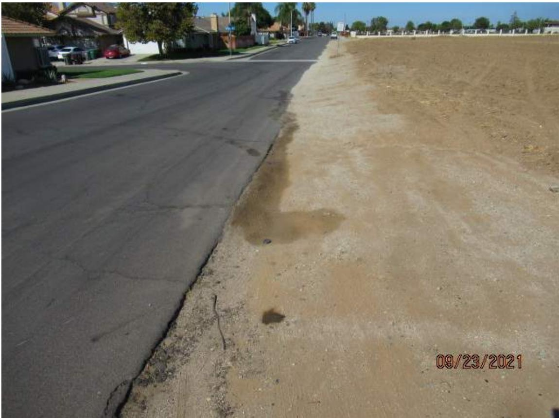
**PHOTO 12** - Westerly view along the north side of the roadway for Copper Cove Lane, showing heavy hydrocarbon-stained soils and asphalt pavement, likely from waste oil. These stained soils are situated within the right-of-way for Copper Cove Lane.
