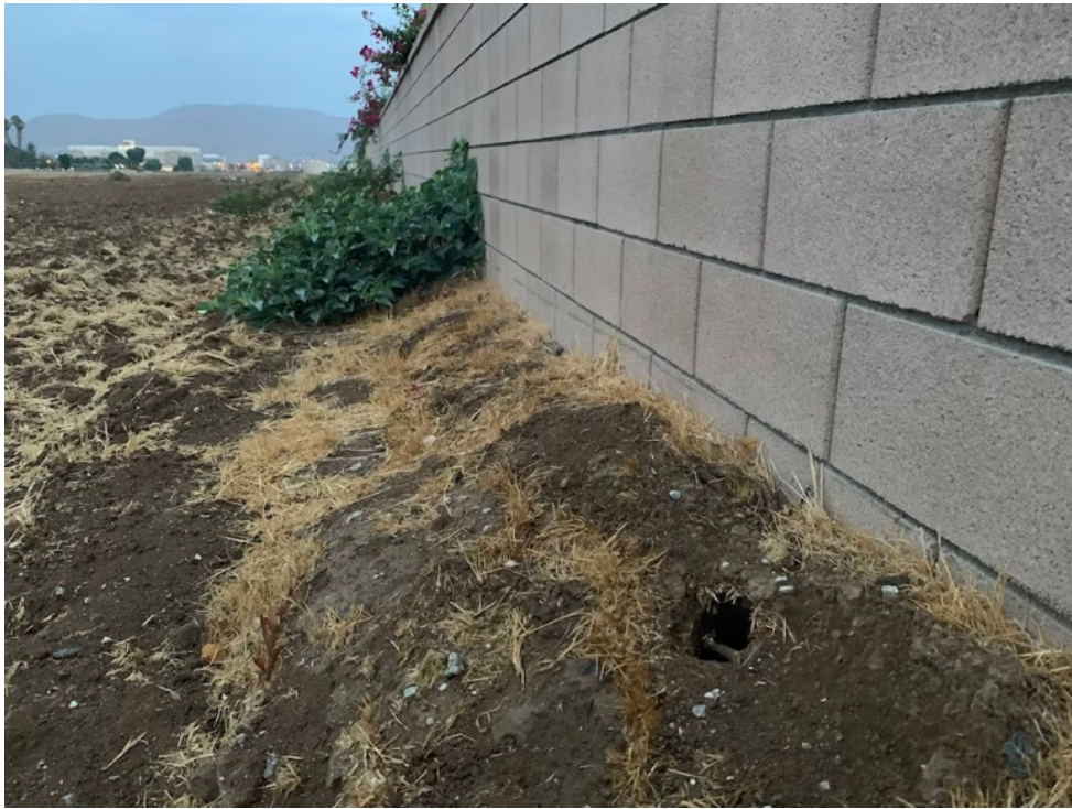
Photograph 7: Representative photo of a suitable BUOW-burrow along western boundary concrete wall.
