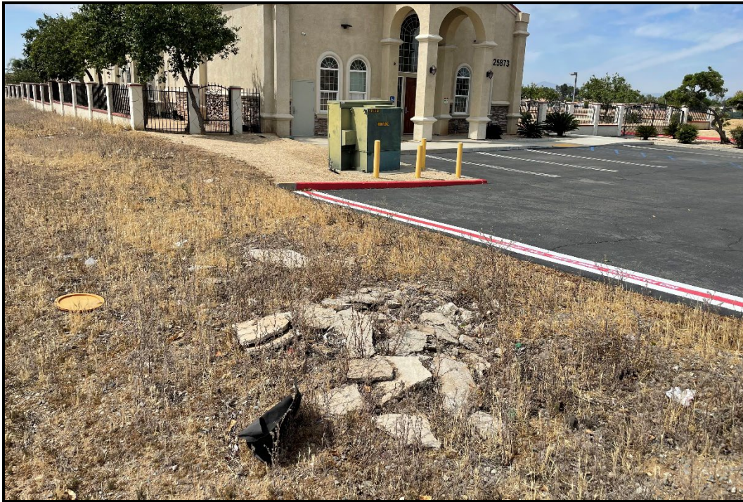
PHOTOGRAPH 3 Concrete Pile Along the Western Edge, Looking Southwest
