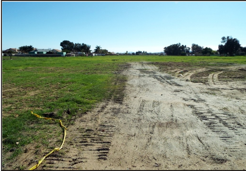
a. Project Overview from Northwest Corner, Looking South (PR-08256-004)
